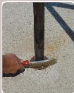
Joints between terrace and the metallic elements (rain pipes, gutters etc), should be clean from dust and rust.
