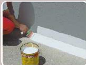
After the primer has dried, **ISOFLEX** or **ISOFLEX-T25** is applied along the intersection in a width of 12 cm approximately.
