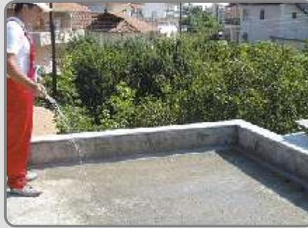
The substrate is dampened, without leaving any water puddles.
