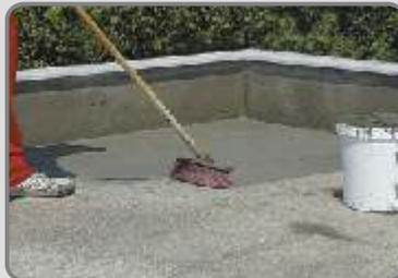
The first layer of **AQUAMAT-ELASTIC** is applied by brush, as wide as the reinforcement (1m). The slurry should be exceeded to the vertical structures (parapet etc) at least 15-20cm up.
