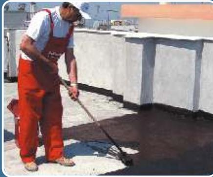
The terrace is primed with the bituminous emulsion **ISOPAST** (diluted 20-50% with water) or with the bituminous varnish **ISOLAC**.
