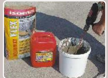
The content of component A (mortar) is added into the liquid component B (elastifying agent), under continuous stirring, until a uniform viscous mixture of **AQUAMAT-FLEX** is formed.
