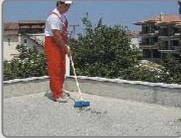
Substrate should be thoroughly cleaned from any loose particles, grease, dust etc.
