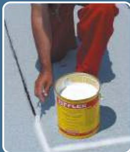
Adjacent membranes should overlap each other at a width of approx. 10 cm. The joints are sealed with a blowtorch and by being pressed with a trowel. Afterwards, **ISOFLEX** or **ISOFLEX-T25** is applied to all joints.
