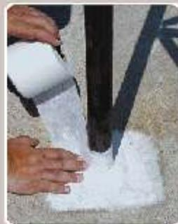
While the first layer of **ISOFLEX** or **ISOFLEX-T25** is still fresh, a glass mesh or polyester fabric strip is positioned.
