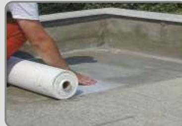
While the layer of **AQUAMAT-ELASTIC** is still fresh, the reinforcing material (**TREVIRA**-1m width) is positioned and embodied.
