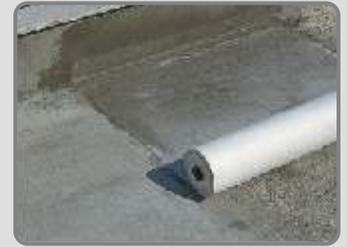
The sheets of reinforcing material should be positioned in sequence so that they overlap each other by 10 cm.
