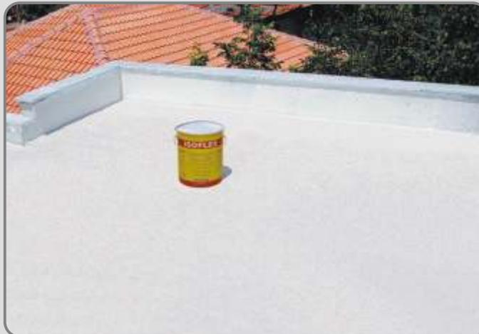
The final result is a uniform, elastic and waterproofing membrane without joints or seams. The main advantage of **ISOFLEX** or **ISOFLEX-T25** is its durability to time due to its composition as a waterproofing material and not as a simple colour.
