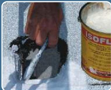
The gutters should be cleaned and then coated with **ISOFLEX** or **ISOFLEX-T25**, reinforced with polyester fabric strip (**TREVIRA**).
