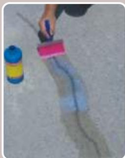
The surface should be dry. Then, the crack is primed along its length and in a width of 12 cm approximately, with the special primer **ISO-PRIMER**.
