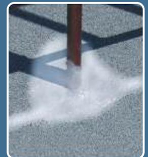
Joints between membrane and the metallic elements (rain pipes, banisters etc), are sealed with **ISOFLEX** or **ISOFLEX-T25**, reinforced with polyester fabric strip (**TREVIRA**).
