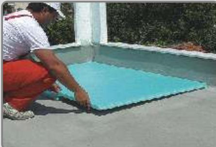
On top of the waterproofing layer and after it has dried out, the extruded polystyrene boards are placed, fixed by their weight.
