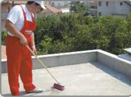
Substrate should be thoroughly cleaned from any loose particles, grease, dust etc.
