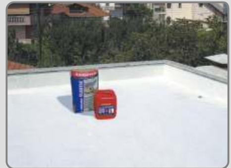
The final layer of **AQUAMAT-ELASTIC** should be white in order to reduce the absorption of heat from the sun's rays and extend the life of the waterproofing.
