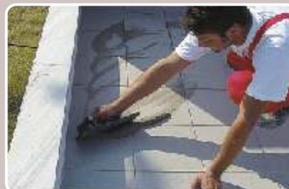
The tile grout **MULTIFILL 3-15** should be reinforced with the polymer-based admixture **DS-99**.
