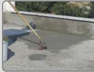
**AQUAMAT-FLEX** is applied over the entire roof surface, in strips of 1 m.
