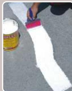
After the first layer of **ISOFLEX** or **ISOFLEX-T25** has dried, two further layers are applied along the cracks.
