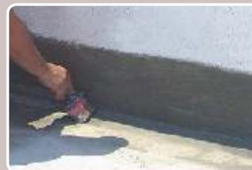
A layer of **AQUAMAT-FLEX** is applied locally, along intersections of terrace with vertical structures (parapet etc.), along possible cracks, tiles and joints between the terrace and any metallic elements (rain pipes, gutters etc). While it's still fresh this layer is reinforced with a **polyester fabric strip (TREVIRA - width 10cm)**. If it is necessary, a second layer of **AQUAMAT-FLEX** is applied, in order to achieve better embodiment of the reinforcement with **AQUAMAT-FLEX**.
