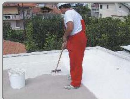
A 3<sup>rd</sup> layer of white **AQUAMAT-ELASTIC** is applied crosswise and once the previous layer has dried. The thickness of each layer should not exceed the 1 mm.
