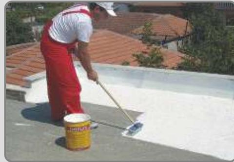
Afterwards, a layer of **ISOFLEX** or **ISOFLEX-T25** is applied with a brush or roller. If it is necessary, **ISOFLEX** or **ISOFLEX-T25** is diluted 5% with water, in order to be applied easier.
