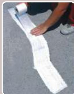
The strips of glass mesh or polyester fabric are positioned while **ISOFLEX** or **ISOFLEX-T25** is still fresh.
