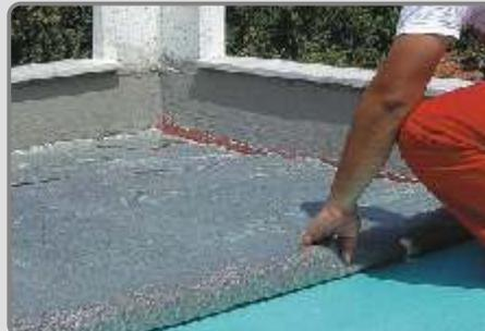
The polystyrene boards are covered with geotextile or plastic linoleum.
