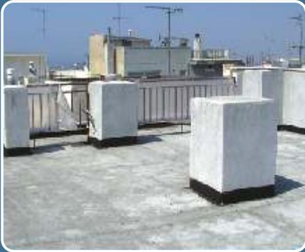
Any necessary repairs to the substrate should be carried out using the polymer-modified cement mortar **DUROCRET**. Bituminous membranes should be laid on a clean and dry substrate.
