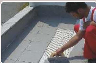
For the adhesion of tiles it is used the 2-component, elastic tile adhesive **Isomat AK-ELASTIC**.
