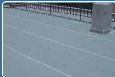
Using bituminous membranes is an ideal solution for waterproofing, as long as the membranes are sealed carefully and the joints with other elements are especially treated. It is recommended bituminous membranes to be placed by professionals.
