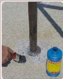
The dry surface is primed with **ISO-PRIMER** all around the joint.
