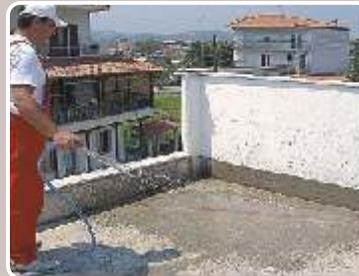
The substrate is dampened, without leaving any water puddles.
