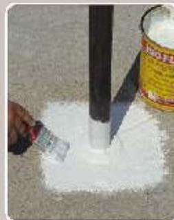
Afterwards, two further layers of **ISOFLEX** or **ISOFLEX-T25** are applied to the joint.
