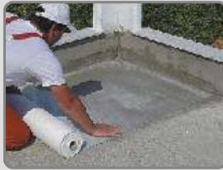
While the layer of **AQUAMAT-FLEX** is still fresh the reinforcing material (**TREVIRA - 1 m width**) is positioned and embodied.
