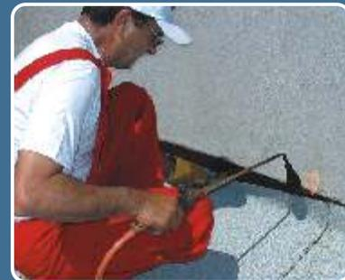
The extensions of membranes to the vertical surfaces (parapets, stairs, termination etc.), are sealed by heating with a blowtorch and then by being pressed with a trowel.
