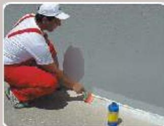
Intersection of the terrace with the vertical structures (parapet, stairwell termination etc.) should be clean and dry. The surface is primed with **ISO-PRIMER**.
