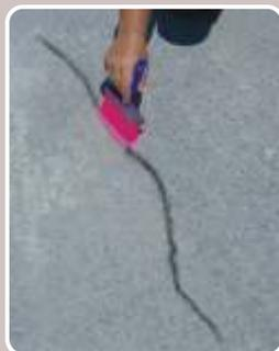
Primarily, there are detected any cracks in the cement mortars, the mosaic or in the old waterproofing layer. Then, any dust or grease, are cleaned.
