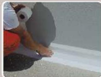
While the first layer of **ISOFLEX** or **ISOFLEX-T25** is still fresh, a glass mesh or polyester fabric strip is positioned from both sides of intersection.
