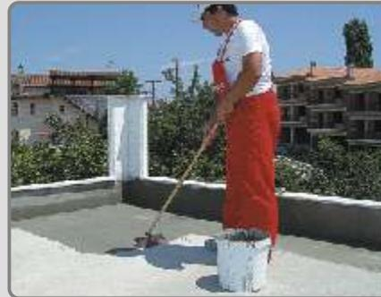
A third coat of **AQUAMAT-FLEX** should be applied crosswise once the previous one has dried. The thickness of each layer should not exceed the 1 mm.
