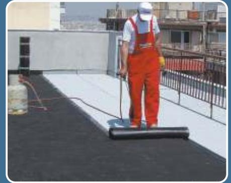
After the primer has dried, the bituminous membranes are heated with a blowtorch and stuck to the surface by simple pressure, starting from the lower points and vertical to the gradients.
