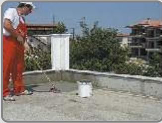
The first layer of **AQUAMAT-FLEX** is applied by brush, as wide as the reinforcement (1m). The slurry should be exceeded to the vertical structures (parapet etc) at least 15-20 cm up.
