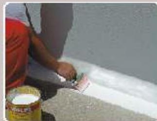
Two further layers of **ISOFLEX** or **ISOFLEX-T25** are applied, each one only after the prior has completely dried.
