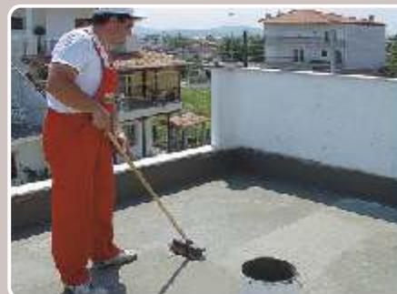
A 2<sup>nd</sup> layer of **AQUAMAT-FLEX** is applied crosswise and once the previous layer has dried. The thickness of each layer should not exceed the 1 mm.
