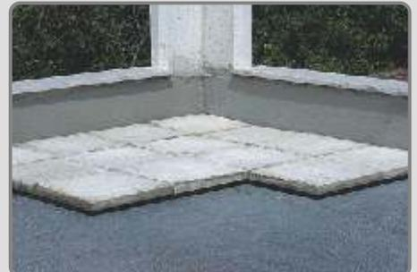
Finally, paving slabs or gravel (6-8 cm thick layer) are placed in order to protect the waterproofing and insulation layers from the sun and the wind. In this way we can also ensure that the terrace can be walked on.
