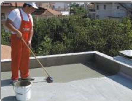
After drying, the reinforced with **TREVIRA** first layer is covered by a second layer of **AQUAMAT-ELASTIC**.
