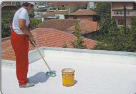
A second coat of **ISOFLEX** or **ISOFLEX-T25** should be applied crosswise once the first one has dried and can be walked on.
