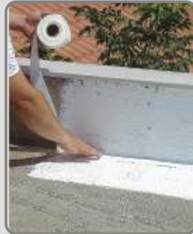
After the primer has dried, a layer of **ISOFLEX** or **ISOFLEX-T25** is applied along the intersection of the terrace with vertical structures (parapet etc.) as well as along any cracks, tiles and joints between the terrace and any metallic element (rain pipes, gutters etc). While it's still fresh this layer is reinforced **with a glass mesh or polyester fabric strip of 10 cm width (TREVIRA)**.
