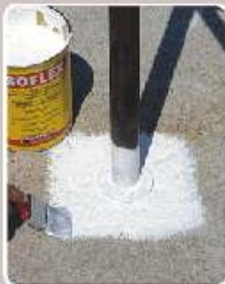
After the primer has dried, **ISOFLEX** or **ISOFLEX-T25** is applied all around the joint, including the vertical element.
