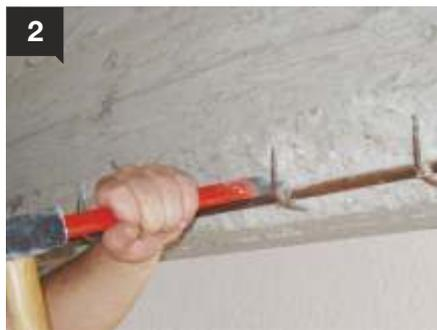
Initially, all broken and loose particles of the peeled concrete should be removed thoroughly, and the corroded steel reinforcement should be completely uncovered.
