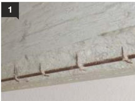
The corrosion in reinforcement, which has led to the detachment of concrete parts, endangers the whole structure.
