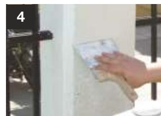
4 The material is applied with a putty knife in one or two layers, depending on the imperfections of the surface. The second layer may be applied, after the first one has dried.
