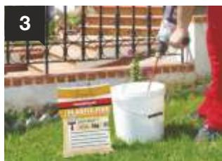
3 The cement putty is gradually added into water, under continuous stirring, until a uniform pasty putty is formed, proper for stuccoing.
