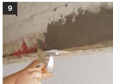
The material is applied by pressure with a trowel.
