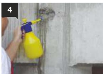
4 Subsequently, the surface is thoroughly dampened.
