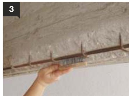
Subsequently, the corroded steel is cleaned and scrubbed, ground etc. with an appropriate tool in order for the rust to be completely removed.
