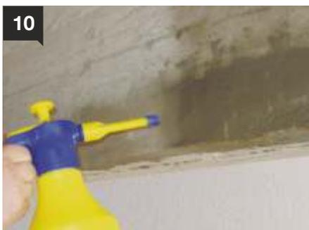
The final surface should be well protected from dehydration for 48 hours, e.g. repeating dampening.
