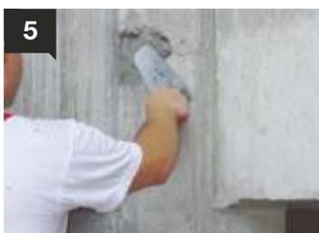
5 The cavity is filled with **DUROCRET**. The material is applied by pressure with a trowel.
