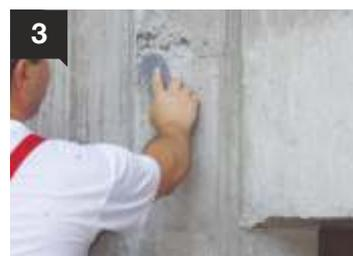
3 Then, it is cleaned of any dust with the use of a hard brush.
