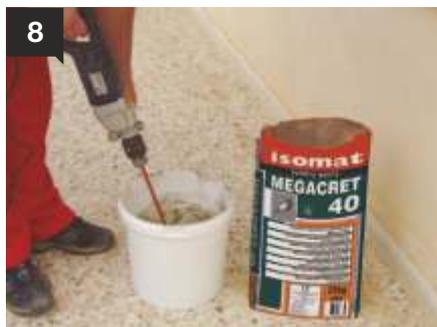
The peeled area of the concrete is repaired with the application of **MEGACRET-40**. Its preparation requires only the addition of water.
