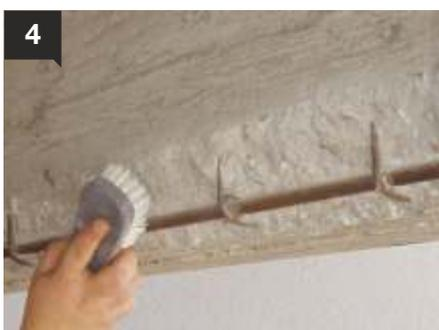
Next, the surface is thoroughly cleaned of any dust.
