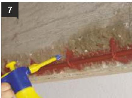
After **FERROSEAL** has dried, the surface is dampened thoroughly.
