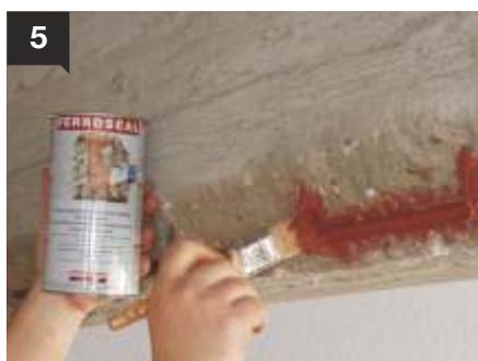
**FERROSEAL** is applied with a brush in two layers. Its preparation requires only the addition of water.
