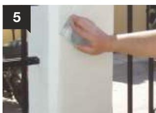
5 After the surface has hardened, it is rubbed with a thin sand paper.
