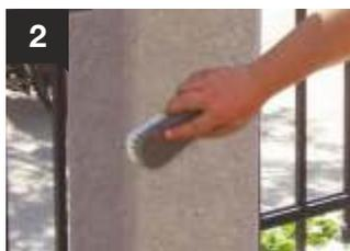
2 Firstly, the surface is cleaned of any dust and is thoroughly dampened.
