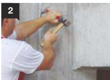
2 Firstly, the surface is cleaned of any loose particles, by mechanical means.
