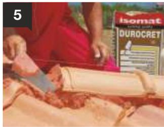
**DUROCRET** is applied with a trowel as usual where the ridge must be placed.
