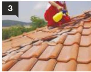
Subsequently, the surface is well dampened.
