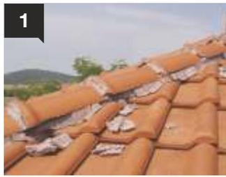
The detachment of ridges is a problem that usually occurs when their fixing is made using a low quality cement mortar.
