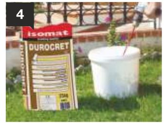
**DUROCRET** (red-brown color) is added into water under continuous stirring, until a mixture of the desired workability is formed.
