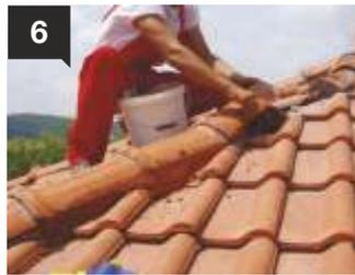
Subsequently, the ridge is fixed and leveled using a thread.
