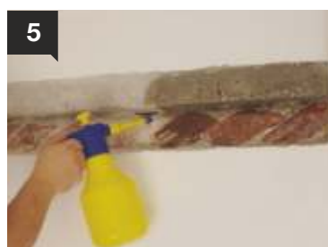
5 Subsequently, the substrate is well dampened.
