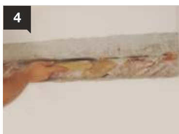
4 The entire area of the detachment is thoroughly cleaned with a brush.
