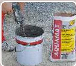
Depending on the water pressure, 2-4 layers of **AQUAMAT** are applied onto the external walls of the basement after dampening. The coating surface must extend at least 50 cm above the ground level. Each layer must be fully dry before the next one is applied. To avoid cracking, each layer should not be thicker than 1 mm.
