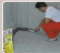
Intersections of the floor with vertical elements (concrete walls, columns), should be dampened and sealed, along their entire length with **DUROCRET** (formation of a "groove"). 2-4 layers of **AQUAMAT** are applied onto the basement floor. The floor coating must extend on the concrete walls or columns at least 50 cm above the groove formed at the intersection with the floor. Each layer must be fully dry before the next one is applied.
