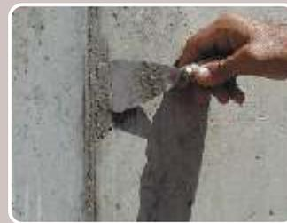
Externally, any cavities in the concrete should be cleaned from loose particles, aggregates etc. Form wires and distance pieces should be cut at a 3 cm depth. Any working joints should be widened in a V-shape along their length, at a depth of 3 cm. The surface of the above areas should be thoroughly dampened and filled with **DUROCRET** polymer modified cement mortar.
