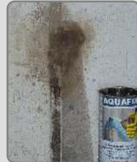
Leaking points are fixed with **AQUAFIX**, a rapid-setting cement for instant sealing of water leaks.
