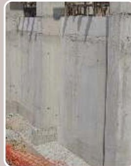
The substrate should be thoroughly cleaned from any possible formwork oil residues, loose particles, dust etc.
