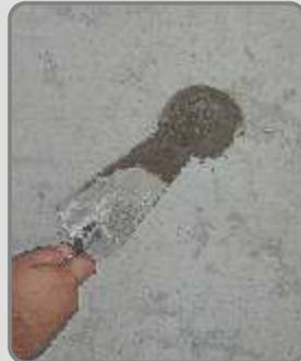
Form wires and distance pieces should be cut at a 3 cm depth. Any working joints should be widened in a V-shape along their length, at a depth of 3 cm. The surface of the above areas should be thoroughly dampened and filled with **DUROCRET** polymer modified cement mortar. Also any cavities in the concrete should be filled with **DUROCRET**.
