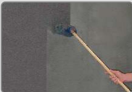
After thoroughly dampening, the walls of basements are coated with **AQUAMAT** on 2-4 layers, depending on the pressure of water. The layer must extend on the concrete walls or columns at least 50 cm above the groove formed at the intersection with the floor. Each layer must be fully dry before the next one is applied. To avoid cracking, each layer should not be thicker than 1 mm.
