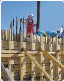
To reinforced concrete it is added **PLASTIPROOF**, a plasticizer, type A concrete waterproofing admixture.
