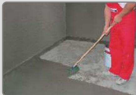
Finally, **AQUAMAT** is applied in the same way to the floor of basement.
