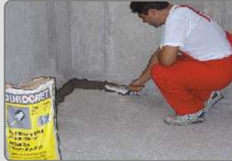
Intersections of the floor with vertical elements (concrete walls, columns), should be dampened and sealed, along their entire length with **DUROCRET** polymer modified cement mortar (formation of a "groove").
