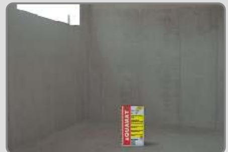
With **AQUAMAT**, a uniform waterproofing layer is shaped in the basement internally. Afterwards, a layer of coat, plaster or tiles can be applied.
