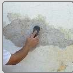
The crumbling particles are removed with a spatula and the surface is thoroughly cleaned from dust.
