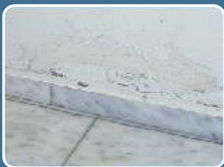
Penetration of water to the intersection between the baseboard and the tile or the plaster has caused bulge and ablation of the colour.
