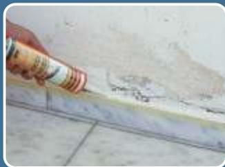
The intersection between the baseboard and the plaster is sealed with **ISOMASTIC- A**.
