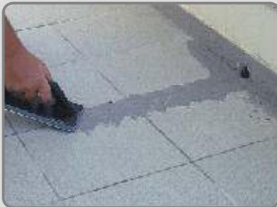
Nextly, the grout should be spread all over the joints with a rubber float in a diagonal direction to the joints, in order to fill them completely.
