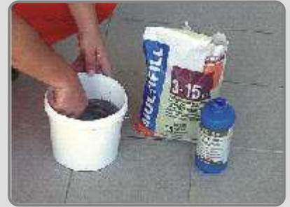
**MULTIFILL 3-15** is added to water under continuous stirring and is reinforced by adding resin **DS-99**.
