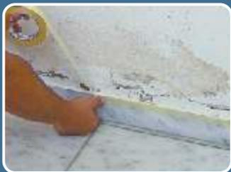
In order to avoid soiling of the adjacent surfaces, the use of adhesive tape is necessary.
