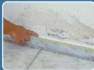
The mastic should be smoothed while it is still fresh and the adhesive tape should be removed straight after.
