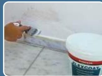
After **ISOMASTIC- A** has dried, the surface is painted with **FLEXCOAT**.
