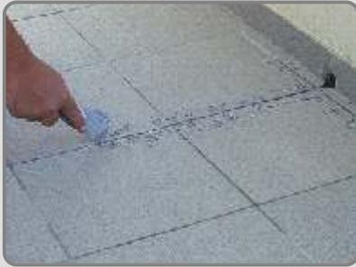
The damaged tile grout should be removed mechanically (spatula, wheel etc).
