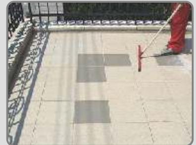
The material is left to act for 5 minutes, next the excessive material is removed using a squeegee.
