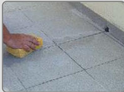
When the grout is dry enough, the surface is wiped with a slightly wet sponge.
