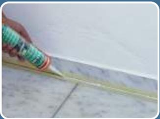
The intersection between the baseboard and the tiles is sealed with **FLEX-PU-40** or **ELASTOTAN**.
