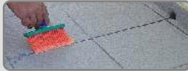
The joints should be carefully cleaned from dust or loose particles and then dampened.
