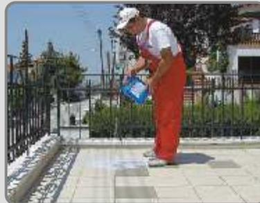
**PS-21** is exuded onto the surface and applied with a squeegee.
