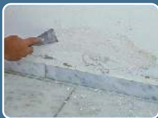
Primarily, the damaged parts of colour are being removed with a spatula.
